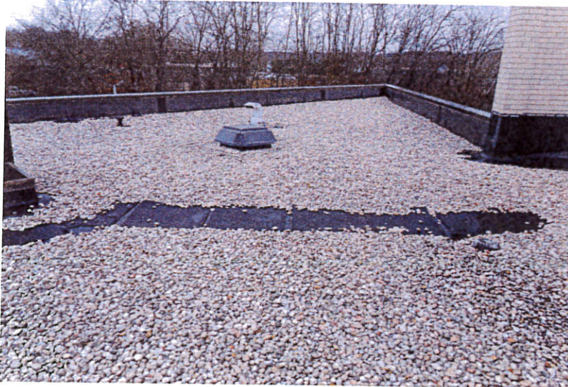
Financial Service Building
